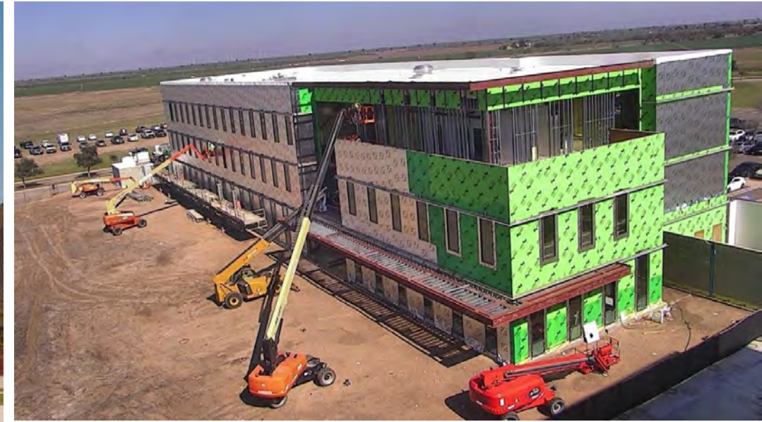
Progress Photo - February 2025
