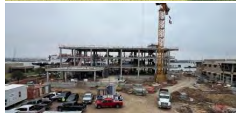
Progress Photo - February 2025
