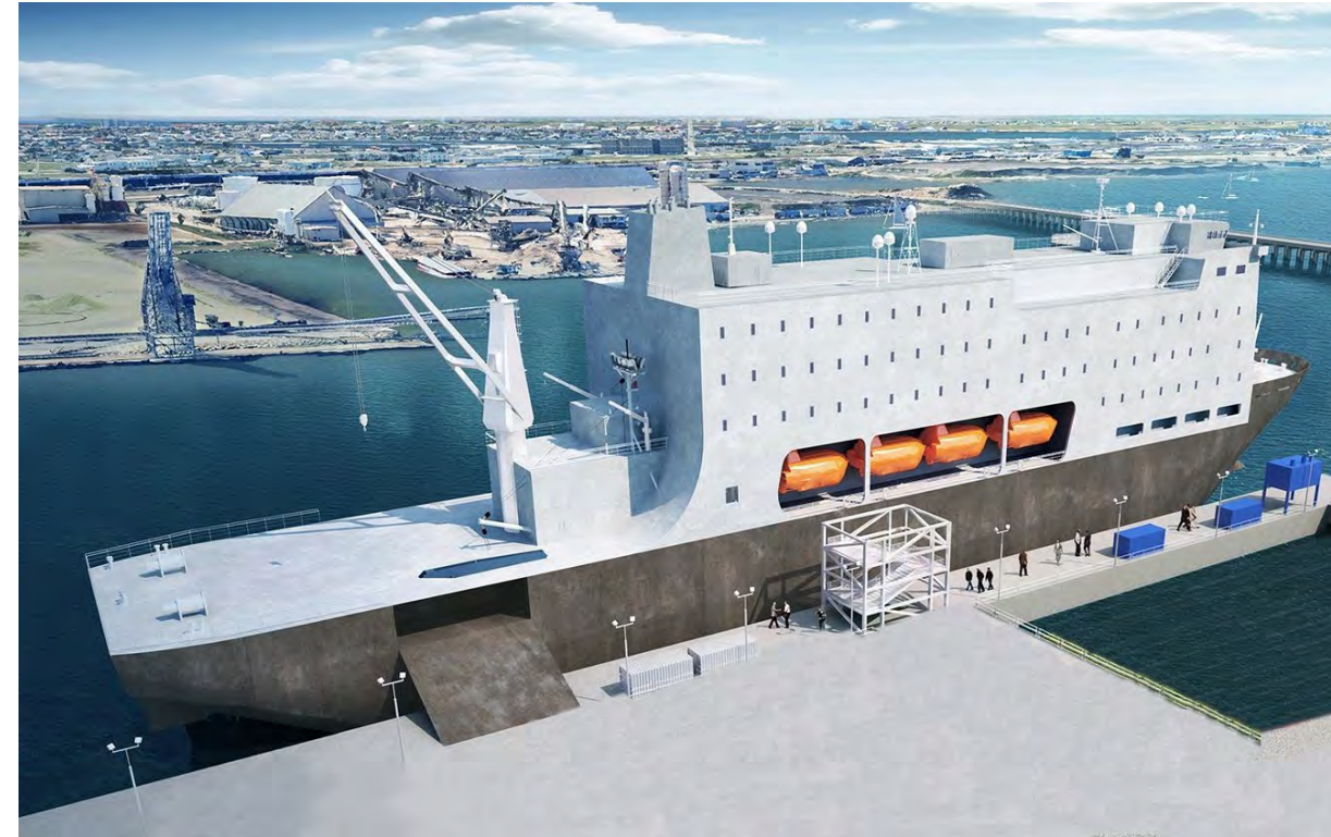
Infrastructure, Dock Improvements, and Ship FF&E – Phase II
