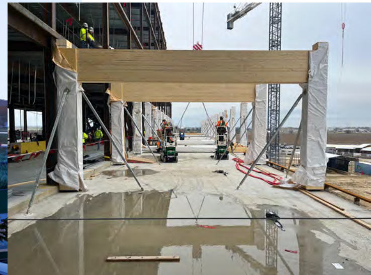
Progress Photos – February 2025
